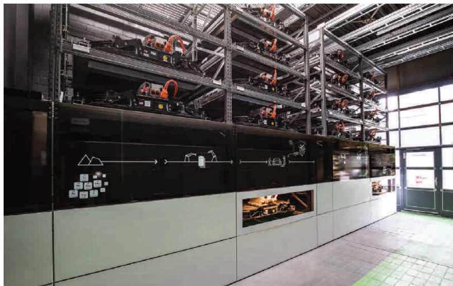
This installation is a demonstration project showing how end-of-life EV batteries can be reused for energy storage.
